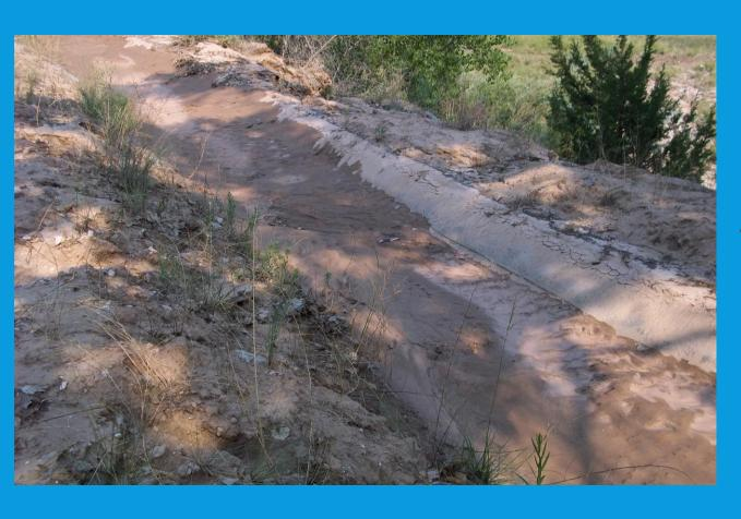
Note the upper left corner of the photo where the acequia is completely covered. The acequia bank on the far side is eroded from the water and mud which spilled over the acequia bank. The bank was completely washed away and the acequia cement liner was hanging in mid-air. Luckily, the cement liner did not collapse.
