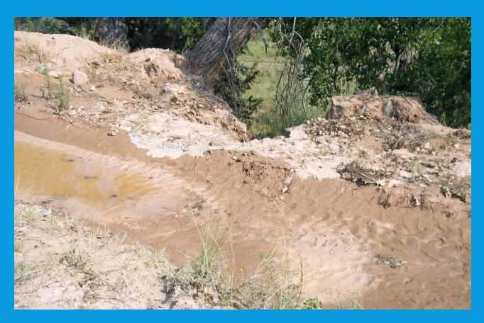
The acequia is in the foreground. It is completely filled-in with mud. The acequia bank is eroded from water and mud spilling over it's side.
