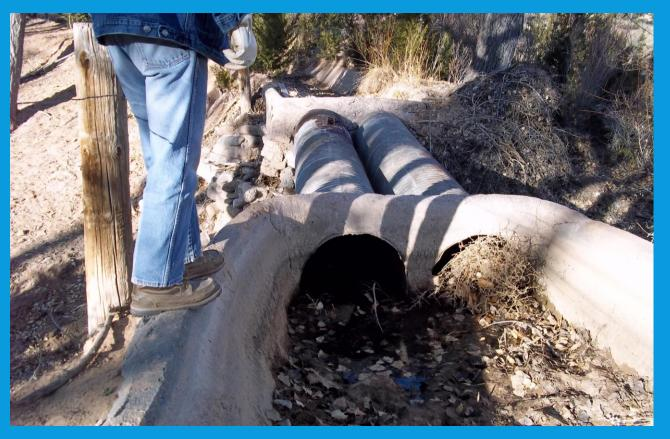
This is the area called the 'Double Canos'. Here the acequia was filled with mud and debris from the 2011 flood. We discovered a desague at this location which had been purposely blocked. Once it was cleaned out, the mayordomo was able to use it to keep the acequia clean.
