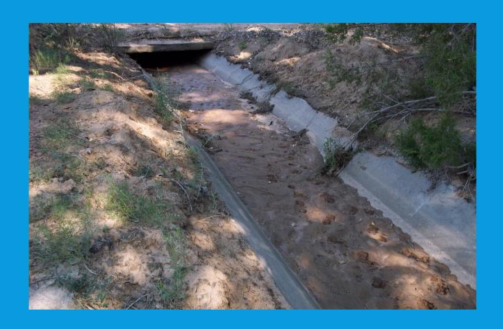
This section of the acequia is partially filled-in with sediment. The bridge seen at the top of the slide is resting on the cement liner.
