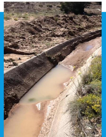
Along with the sediment in the acequia from the 2013 flood, notice the piles of dirt on the acequia bank. Dirt piling up along the acequia bank is becoming an ever increasing problem. Our by-laws state that our members are responsible for keeping their acequia sections free of trash and other obstructions (Article 6, Section 1)
