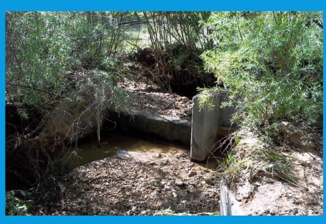
This is the acequia's first, and probably the most crucial, desague. In the 2011 flood, the desague was filled with mud, rock and debris. This desague is a few hundred feet from the presa (diversion) on the Santa Cruz River. The river brings large amounts of sand into the acequia during normal operation, so functioning desagues are critical.
