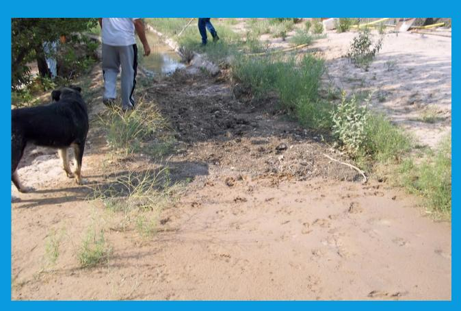
The acequia can be seen at the top of the slide, between the two men. The acequia is also in the foreground, completely covered by sediment. At this location, an arroyo is responsible for the filling in the acequia.
