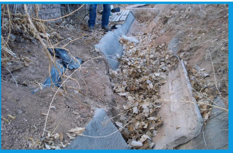
This is an area where the cement liner is broken in several places. There are other areas along the acequia where the cement is broken. There is a large cottonwood tree along the acequia which may have caused the liner to break.
