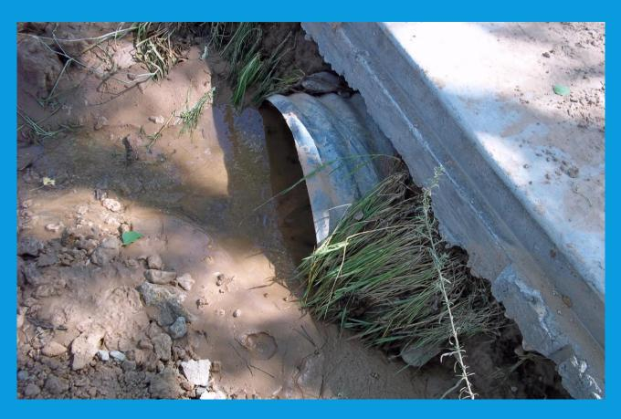
The acequia is filled with sediment from the 2011 flood. The acequia is a dirt ditch in this location. Two brothers cleaned this cano which was packed with rock and mud. It took several hours to complete the job.
