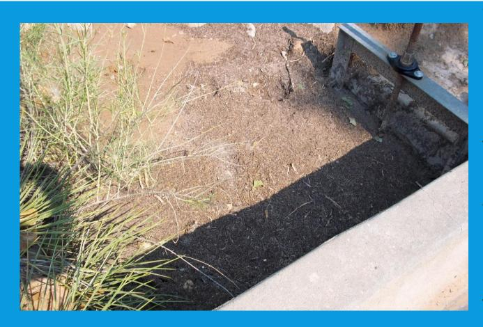
This desague is filled to the top with mud from the 2011 flood. Santa Fe County helped clean the acequia and the desagues and they also reconstructed the eroded acequia bank. SFC worked for several weeks on the acequia. One parciante rented a track hoe, at his own expense, and cleaned the parts of the acequia. Much of the cleaning was done by hand.
