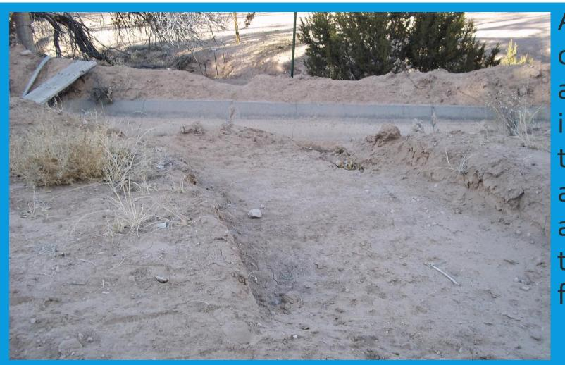
An individual has channeled run-off into the acequia. The Mayordomo is frequently monitoring the acequia for issues such as these. Some individuals are not parciantes, yet they interfere with the functioning of the acequia.
