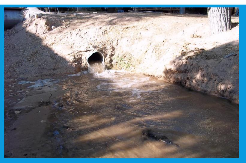
This is the acequia's second desague. It is in a strategic location and it is very important to keep this desague open and functioning properly. The acequia is flushed into an arroyo which runs to the Santa Cruz River.
