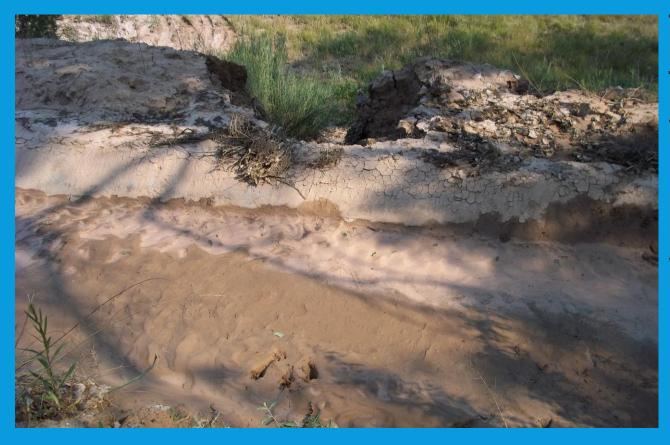
The acequia's bank has eroded from the intense flow of mud and water. Note the steep drop on the eroded side of the bank. This drop-off is approximately 20 feet. With the bank eroded, the acequia was literally suspended in air. Thankfully, the cement liner held; if it would have broken, we would have had a major problem.
